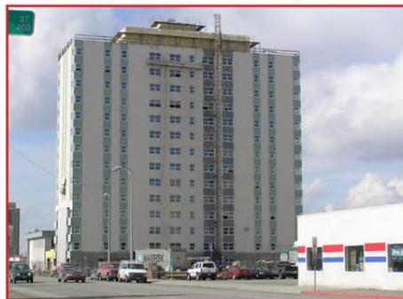
Figure 5: View of nearly-complete and painted building
